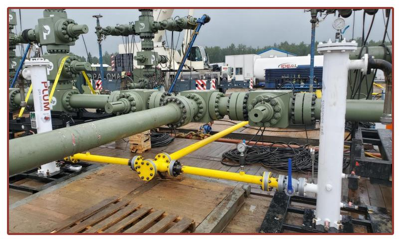
Plum can provide custom supply and distribution manifolds for completions projects designed to provide safe, leak-free fuel gas distribution. Plum manifolds are manufactured in our Drayton Valley, Alberta shop with has its ABSA Certificate of Authorization for B31.3 Process Piping.
